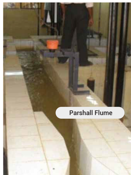
Sewage Treatment Plant
