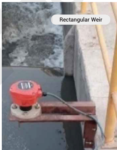
Effluent Treatment Plant
